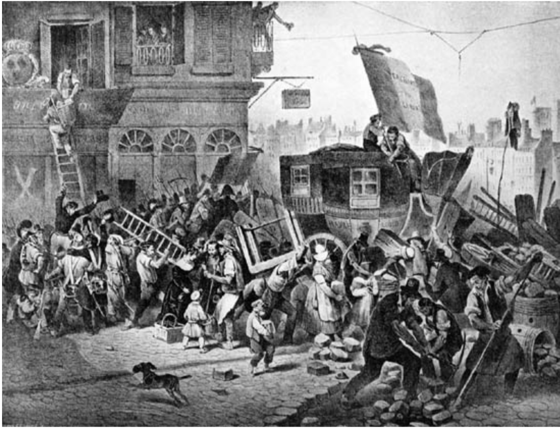
FIGURE 26. Barricade construction in Paris, July 28, 1830. Dayot [1897] n.d.), pt. 1, 33.
